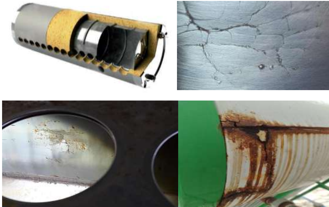
Figure 10: Corrosion phenomena solar thermal equipment.
