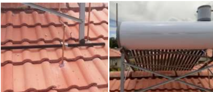
Figure 4: Missing insulation on the copper hot water pipe.
