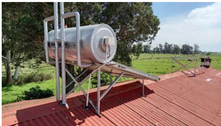
Figure 6: Protection of the insulation material using a weather-proof material that is not susceptible to bird damage.
